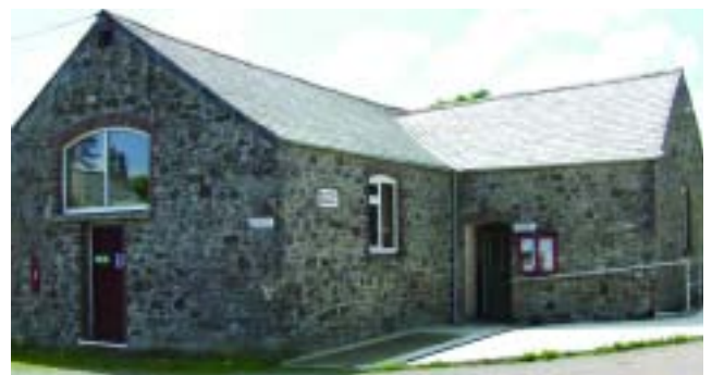
Kelly Village Hall: New level and firm entrance plus accessible parking bay
